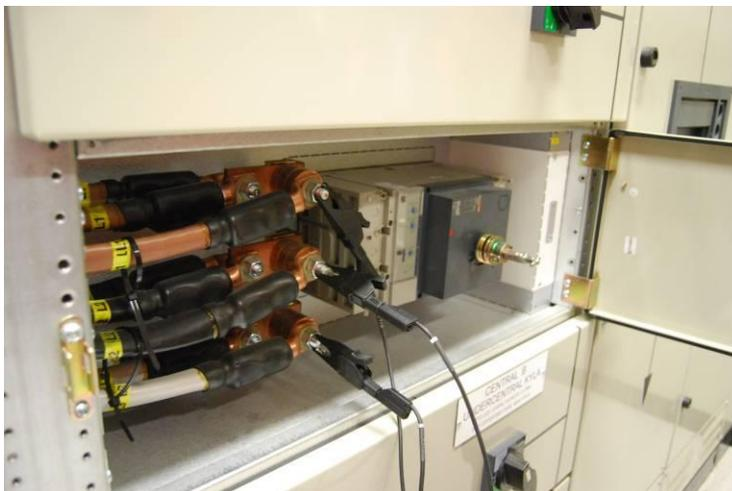
**Figure 4. Mounting of voltage probes of a mobile meter in the electric central signal box.**
